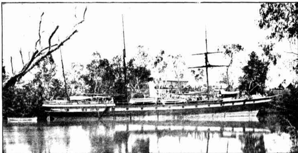
THE TARARUA AT ROPER JETTY.
